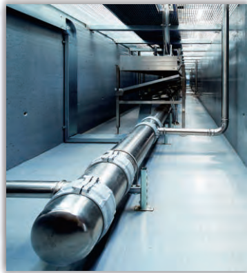
● Koelwater (DN250)
