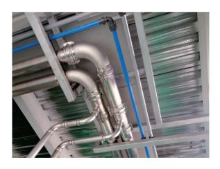
This is a famous auto parts manufacturer, AQUApipe DN25-DN125 for circulating water in production line and injector workshop, blue AIRpipe DN25-DN63 for compressed air.
