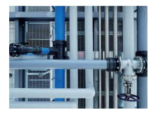
A food packaging enterprise, blue AIRpipe DN20-DN200 for compressed air, gray AIRpipe DN40-DN200 for vacuum. AQUApipe with EPDM seal DN20-DN150 for process water/ hot water/ cooling water, AQUApipe with FKM seal DN25-DN100 for die coolant/ oil.
