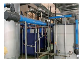
A world leading video-centric smart IoT solution and service provider. AQUApipe DN20-DN200 for cooling water in production line and circulating water in compressor room, AIRpipe DN20-DN125 for compressed air.
