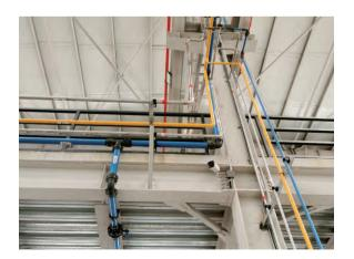
A company specializing in the production air conditioning refrigeration equipment, blue AIRpipe DN25-DN80 for compressed air, AQUApipe DN25-DN50 for propane and oxygen.
